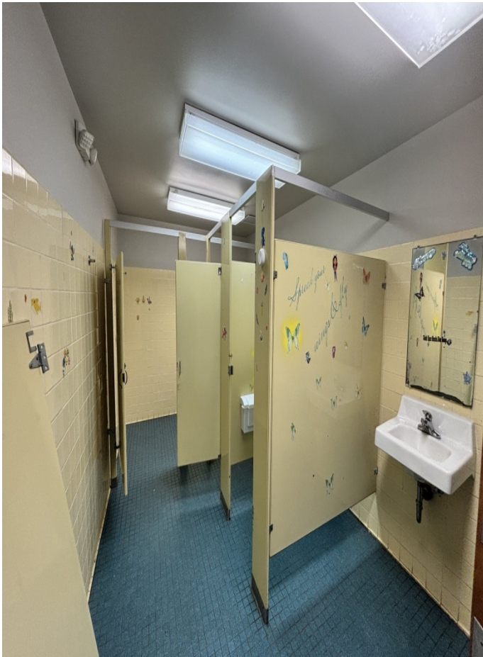
Existing restroom partition configuration.
