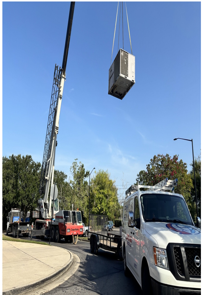
Replacement rooftop HVAC unit being positioned.
