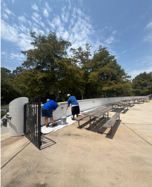
Painting work in progress along the shared wall.
