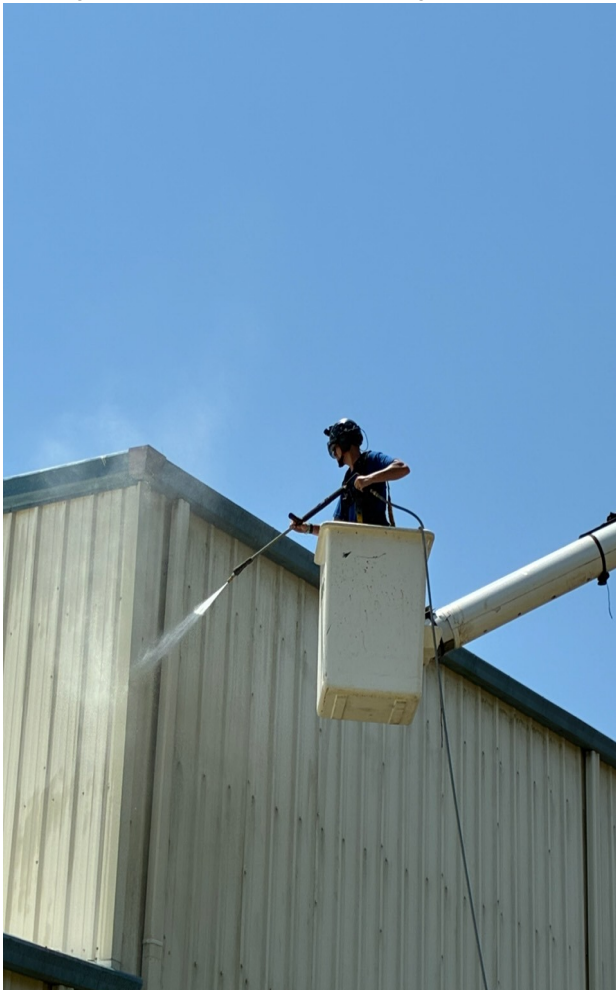
Exterior wall cleaning in progress.
