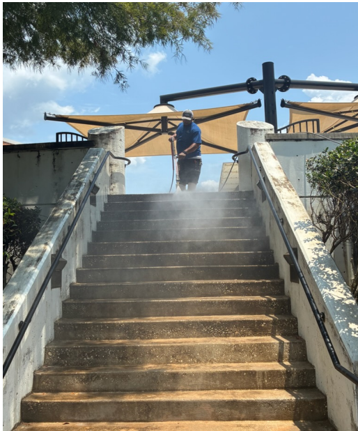
Pressure washing of the exterior stair and wall area.
