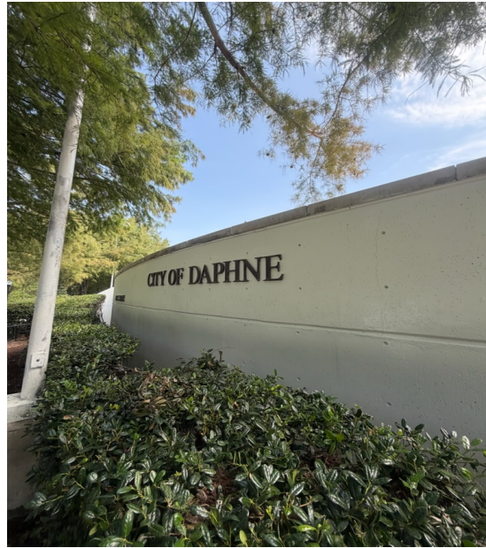
Completed exterior wall with refreshed finish and City of Daphne signage.
