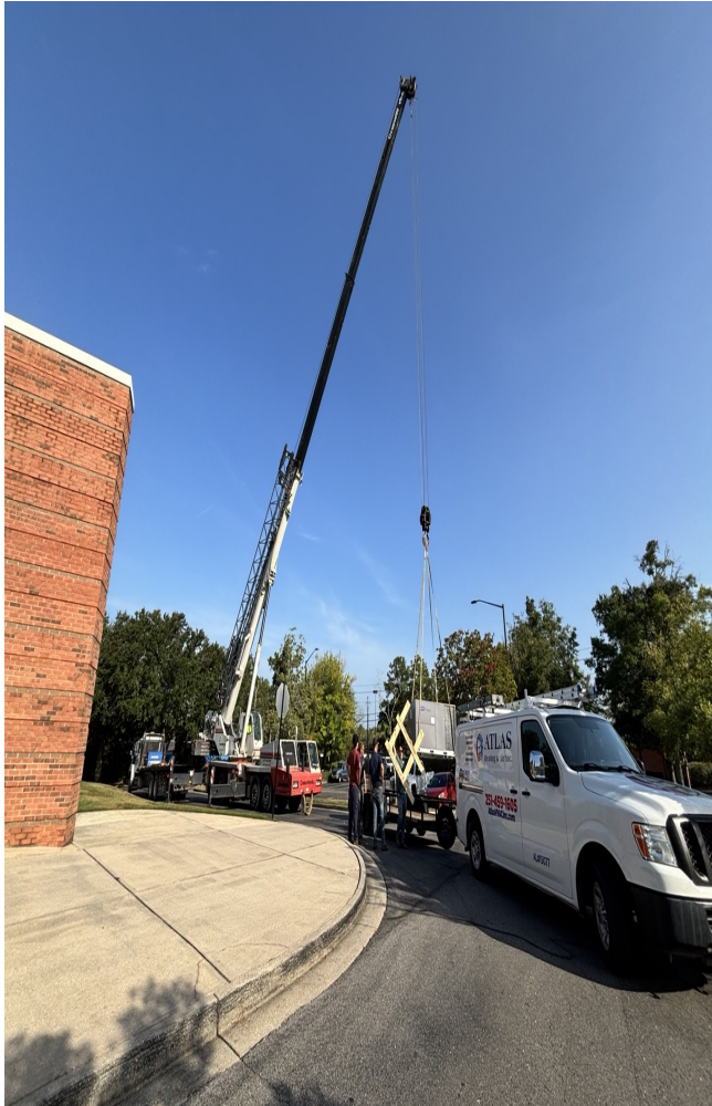
Crane operation supporting rooftop HVAC replacement.
