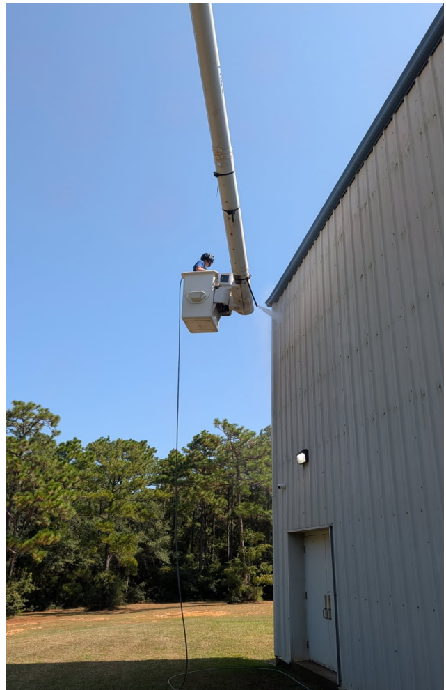
Elevated-access pressure washing of the facility exterior.
