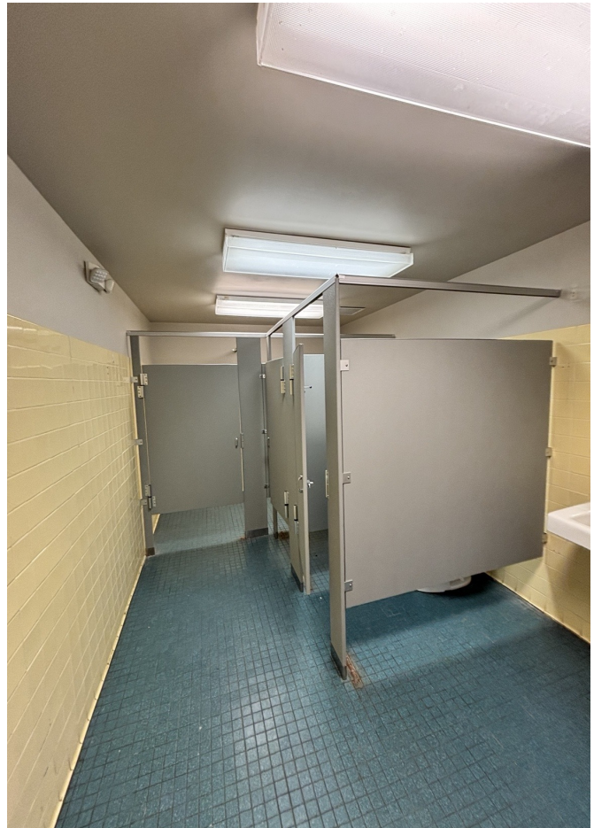
Replacement restroom partitions installed.
