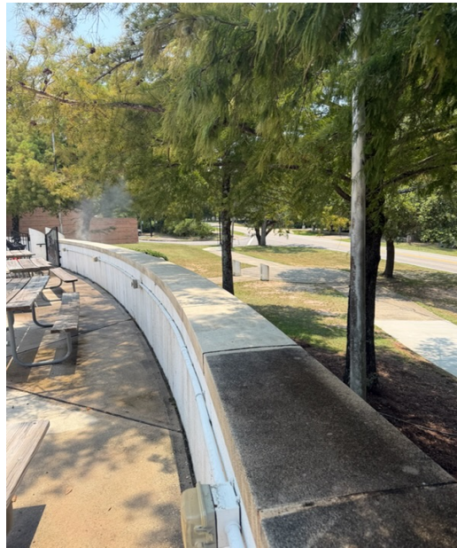
Exterior wall and adjacent public area before/under restoration.
