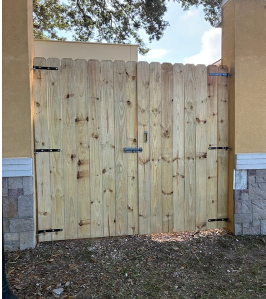
Replacement gate installed at the City Hall generator enclosure.
