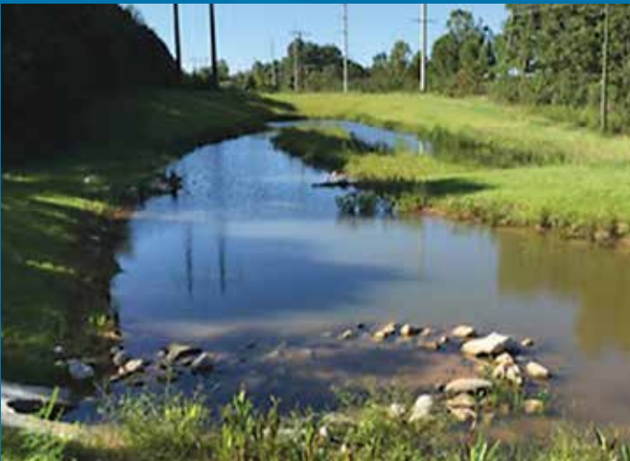
JB SW Management Pond upstream of segment JB at Westminster Village.
