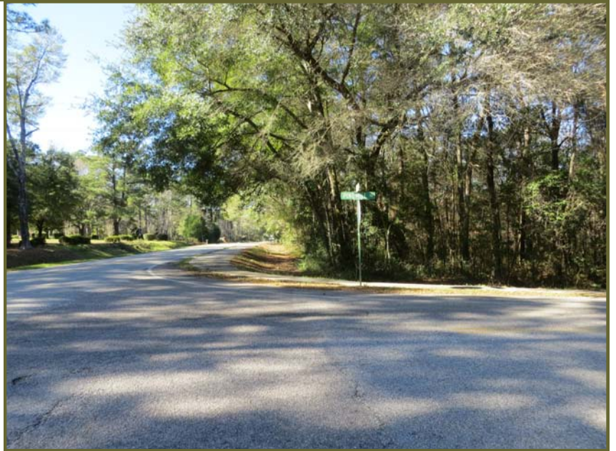
Photo #17 (Right): terminus of the project - intersection of Park Drive - Note: existing sidewalk at this location - new sidewalk will tie into existing
