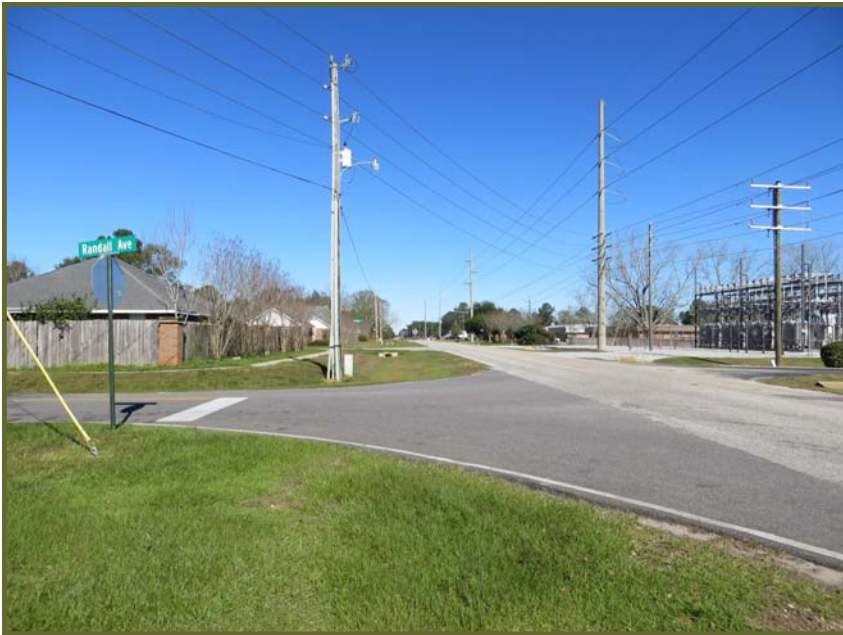
Photo #4 (Left): looking north on Pollard Road at Randall Avenue - Note: Sidewalk at Randall
