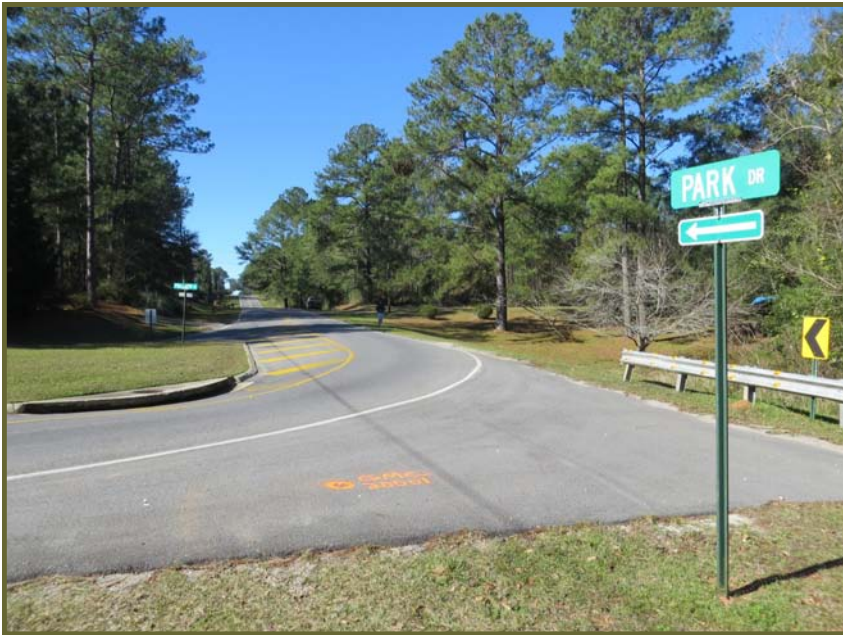
Photo #13 (Left): looking west from Pollard Road along Park Drive
