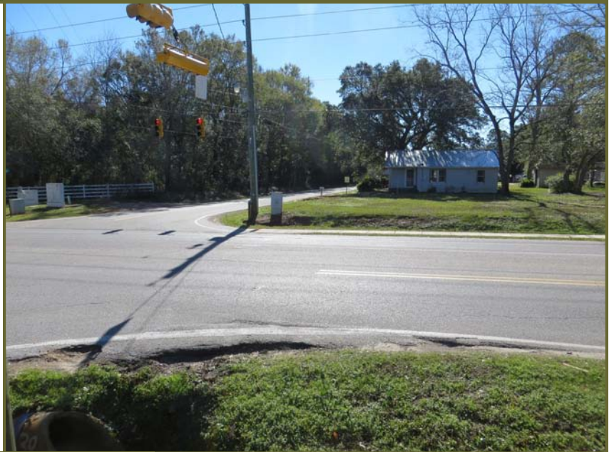
Photo #2 (Right): Looking South at the intersection of County Road 64 and Pollard Road - Start of Project - Note: Sidewalk on south side of CR64
