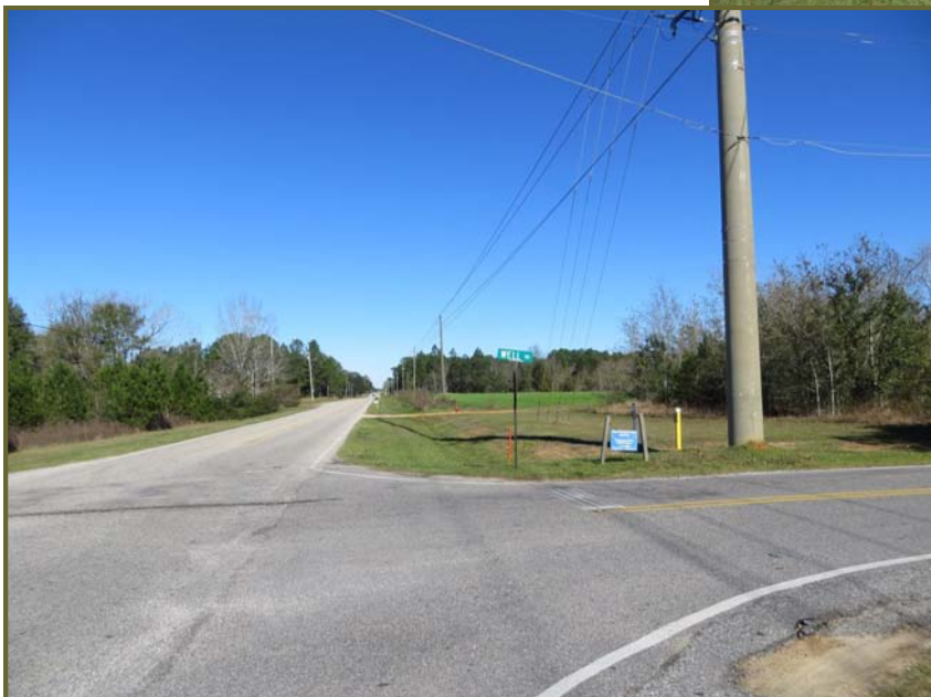
Photo #6 (Left): looking north along Pollard Road from Well Road (east side of R.O.W.) Possible location of a mid-block crossing.
