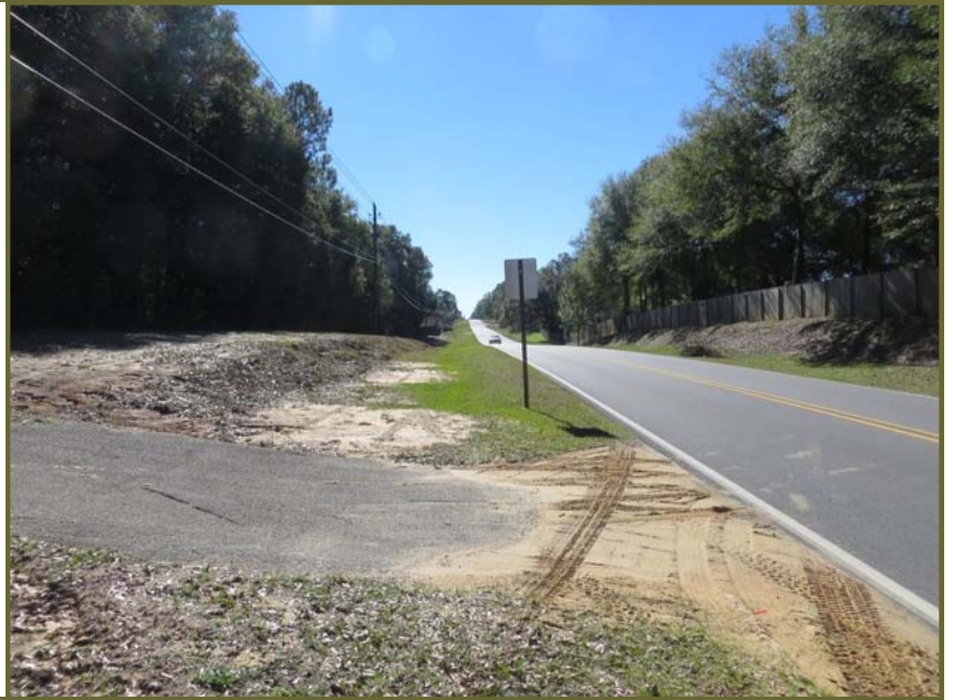
Photo #11 (Right): looking south on Pollard Road along the east side of the R.O.W.
