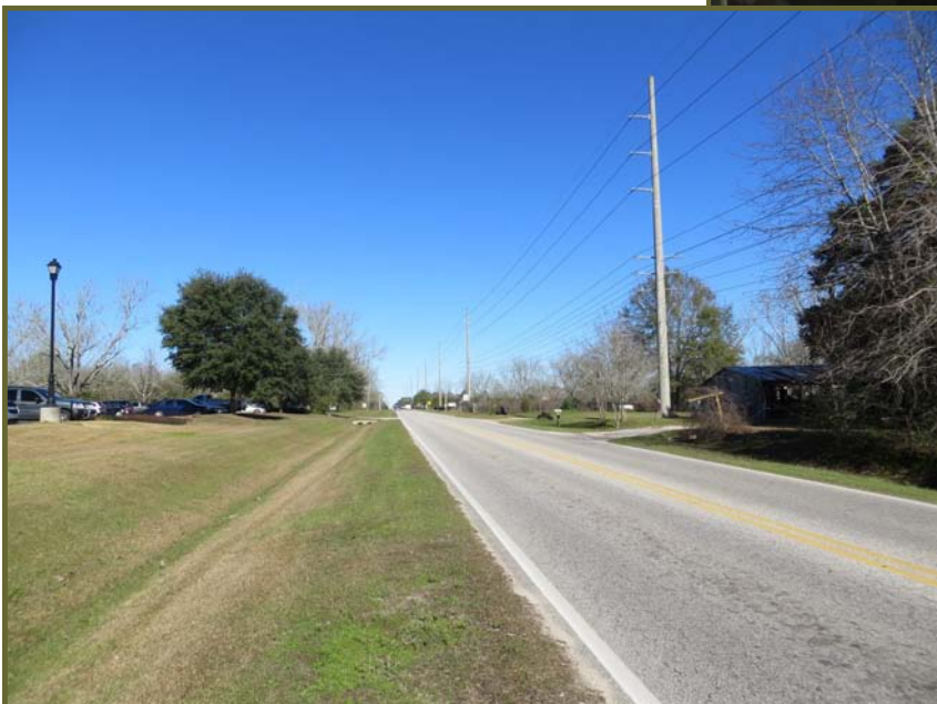
Photo #3 (Left): Looking North along Pollard Road – North of the start of Project (looking towards Randall Avenue)
