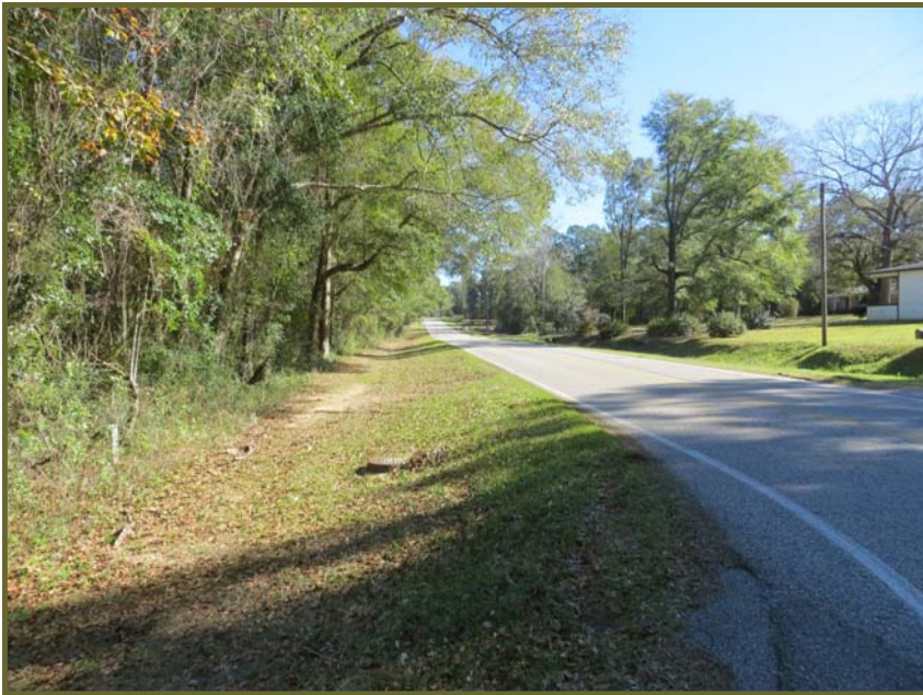
Photo #16 (Left): looking back east along Park Drive (north side of R.O.W.)
